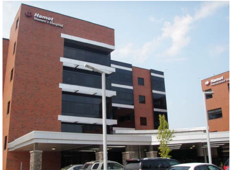
Figure 3: Exterior Building Façade
